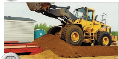
3 Backfill to bulkheads and finish ramps.
