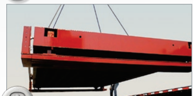
2 Unload and set modules.
